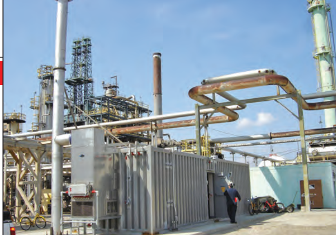
FIGURE 1. Blast-resistant modules like this provide protection for personnel in the event of an onsite explosion
